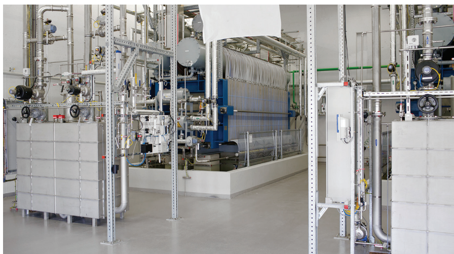
FIG. 1. It is beneficial to work with a trusted central partner across the entire H 2 fuel value chain.
