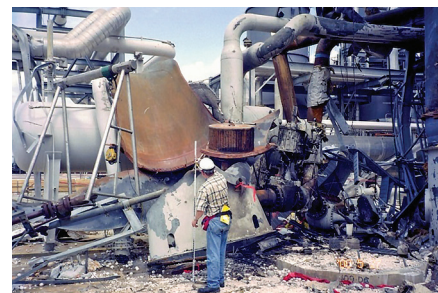
FIG. 3. Brittle fracture of a pressure vessel in an ammonia plant.
